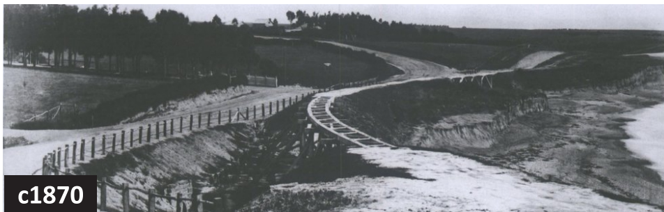
Evans Street and the Rail viaduct under construction. Note the cliff and shore below.
